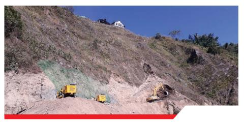
of the collapsed slope and at the same time widens the road bench without increasing the dead load on the slope significantly.
