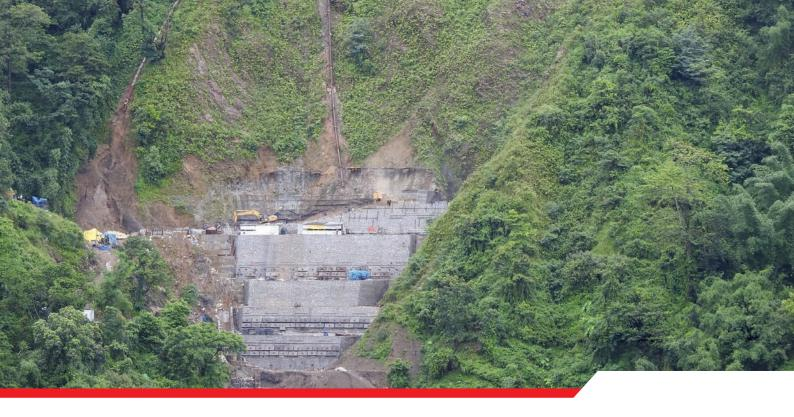
presence of natural aquifer. Therefore, while drilling the holes for nail, significant water flow was encountered. Long semi-perforated pipes were installed within the slope to cater to this challenge.
