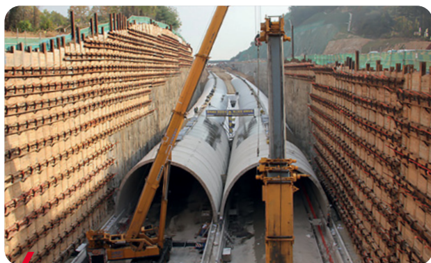
Suwon-Kwang Myeong Motorway (SKM) tunnel, South Korea
