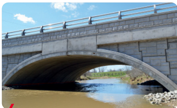
Regional road 14, Canada
