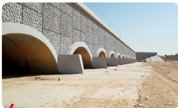
Wadi Stormwater Bridge, Saudi Arabia
